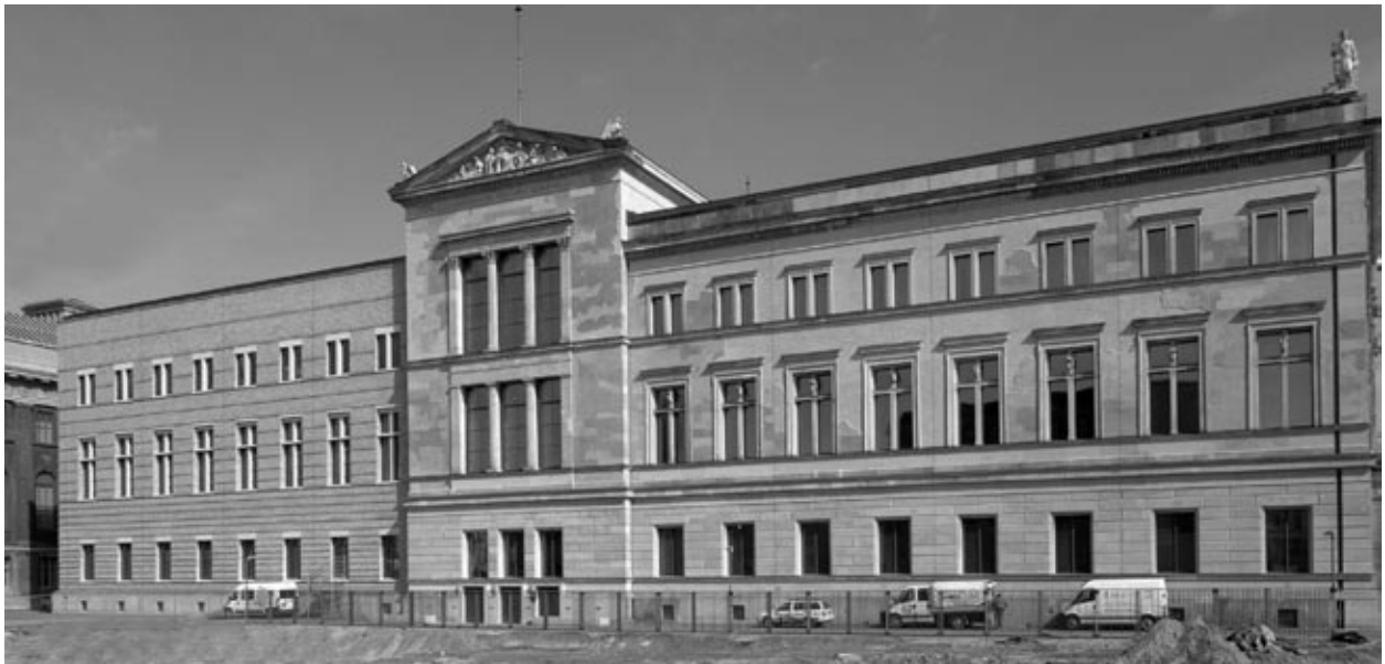
11. Friedrich August Stüler: Neues Museum, 1843 – 1846, Berlin, after the repair by David Chipperfield, 1997 – 2009. Photo: Wolfgang Bittner, Landesdenkmalamt Berlin.
