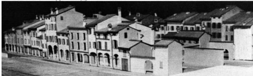
9. Pier Luigi Cervellati (with Roberto Scannavini): Plan for social housing historic center of Bologna, 1972 – 1973, block S. Leonardo, axonometric sketch and view of the model from Via S. Apollonia. Repro: Bologna: politica e metodologia del restauro nei centri storici . Eds. P. L. CERVELLATI – R. SCANNAVINI. Bologna 1973 (2 nd ed.).
