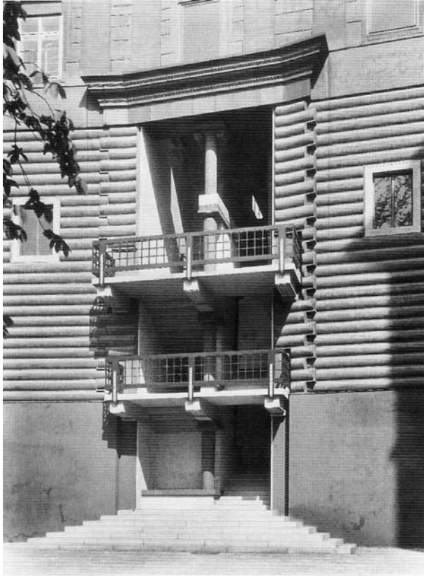
6. J. Plečnik: The Bull Staircase, Prague Castle, 1929 – 1931 . Repr.: LUKEŠ – PRELOVŠEK – VALENA 1996 (see in note 4), p. 281 above.
