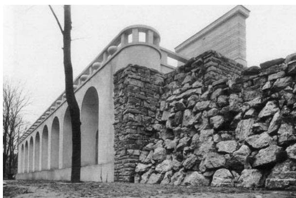
13. J. Plečnik: Access to the Deer Moat, Prague Castle, 1932 – 1933. Repr.: LUKEŠ – PRELOVŠEK – VALENA 1996 (see in note 4), p. 309 above.
